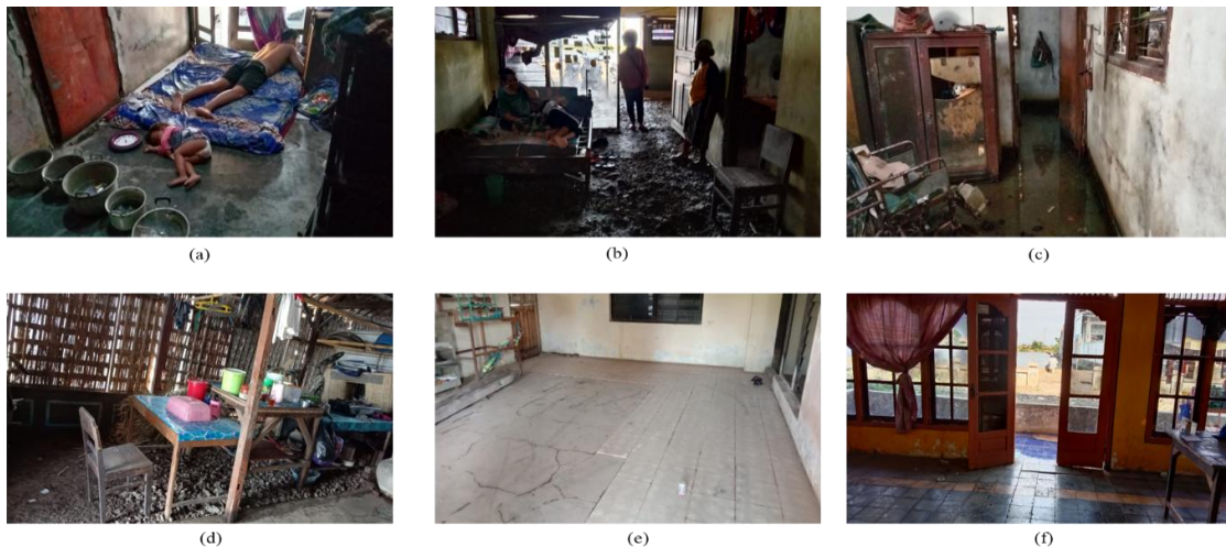
Figure 4. Condition entire house Blacanan Village
