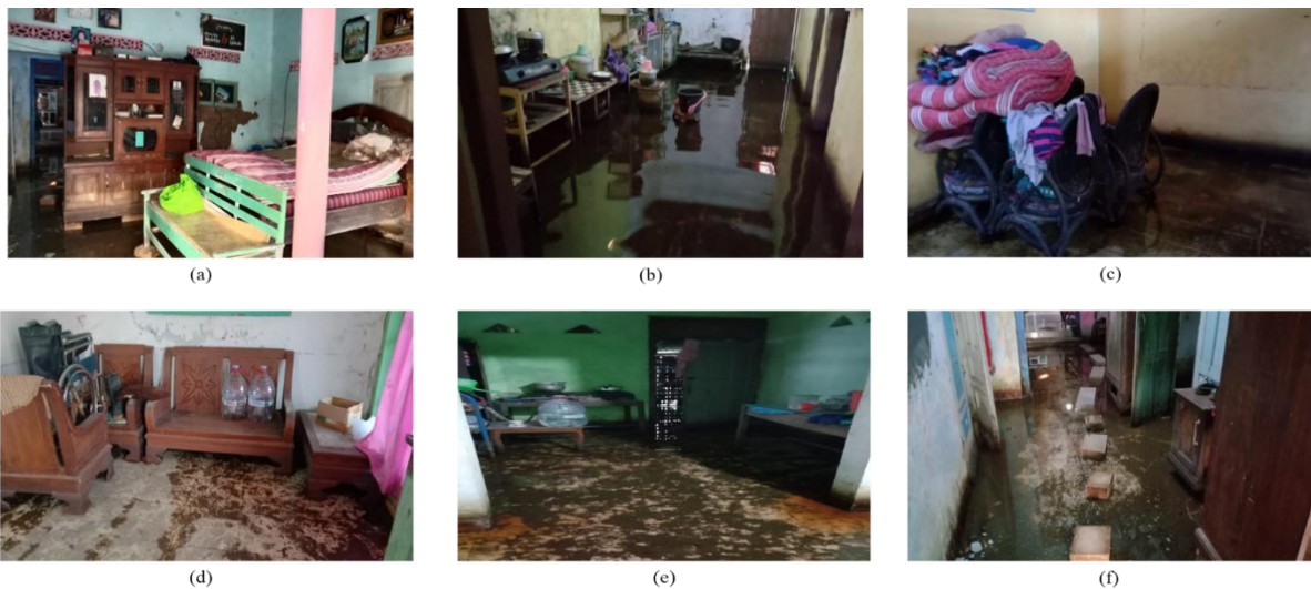
Figure 3. Conditions Entire The House Depok Village
